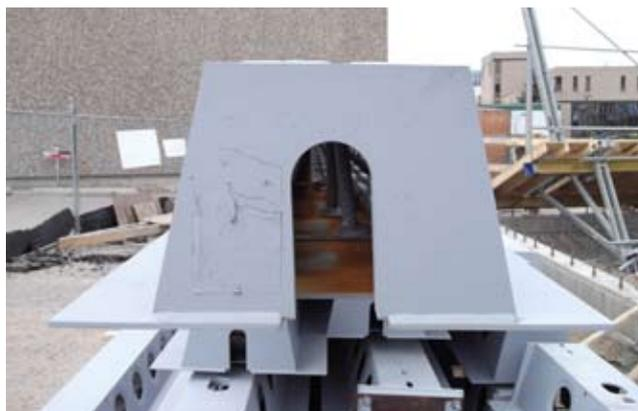
▲ **Three photos, above:** The key to the Deltabeam's quick erection is the end connection. One piece of the corbel is welded to the steel column in the fabricator's shop. The second piece is bolted to the first and provides vertical adjustment. Grooves on the interfacing surfaces maintain the connection's high capacity. The slotted plate welded to the end of the Deltabeam slips over the corbel and the connection is done.
