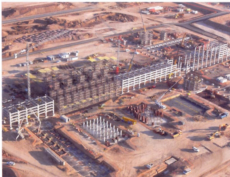
Fig. 1: Overall view of the construction site
