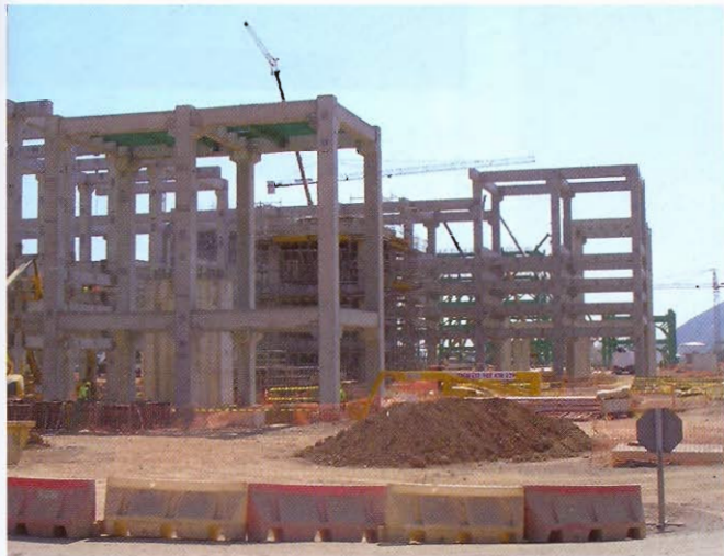
Fig. 3: Pipe rack structure under construction
