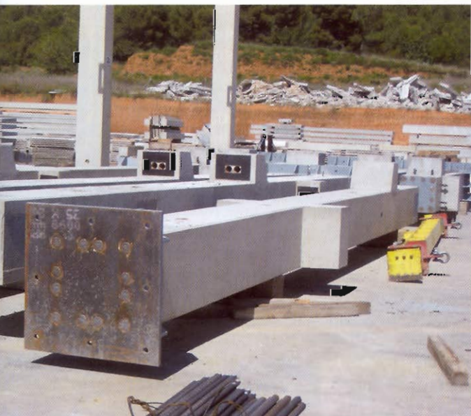
Fig. 4: Multistorey column featuring special steel base plate
