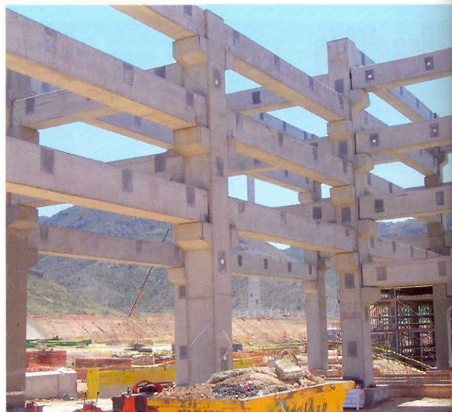
Fig. 2: View of precast concrete pipe rack structure
