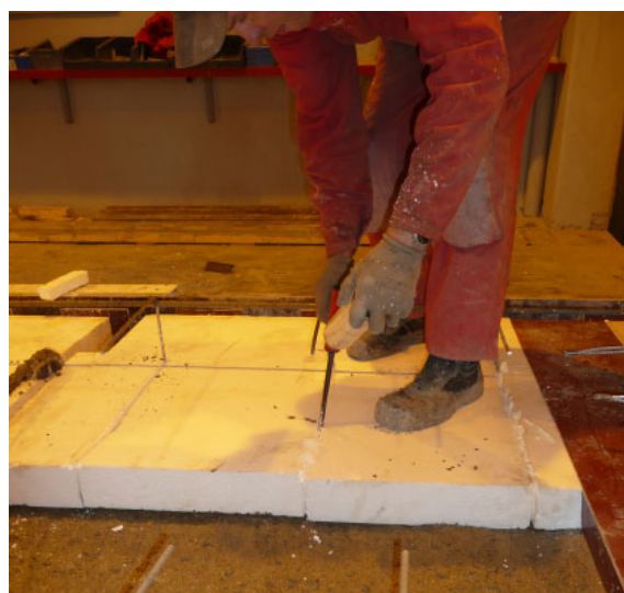
Figure 21. Filling the gaps of hard insulation.
