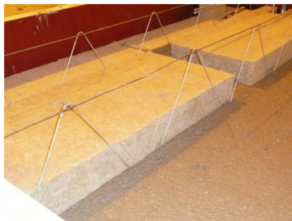
Figure 21. Filling the gaps of hard insulation.
