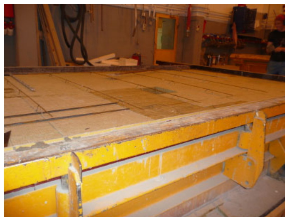
Figure 23. Concrete cover of Diagonal Ties in the inner layer.
