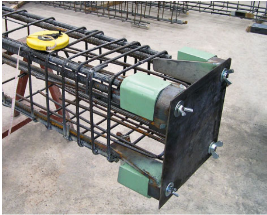
Figure 3. HPKM Column Shoes fastened to mold's plate.
