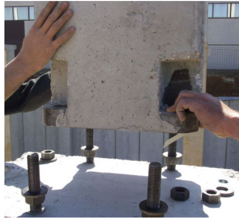
Figure 6. Axial and bending resistance of HPKM Column Connections based on Eurocode 2.
