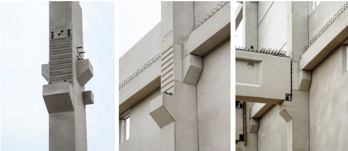
Connecting a COPRA Anchoring Coupler with a BECO Beam Shoe with the help of a threaded bar step by step.
