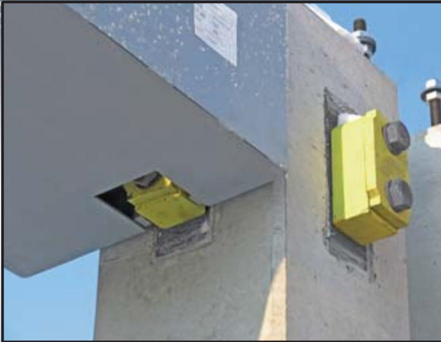
Figure 2: Composite beam supported by PCs Corbels
