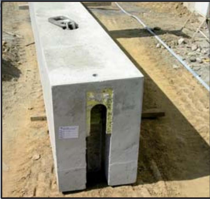
Figure 4: RC beam equipped by PC end plate
