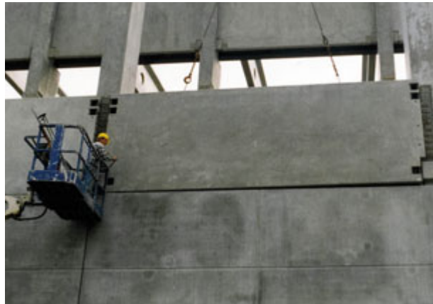
Fig. 4: Vertical joint of a stiffening wall
