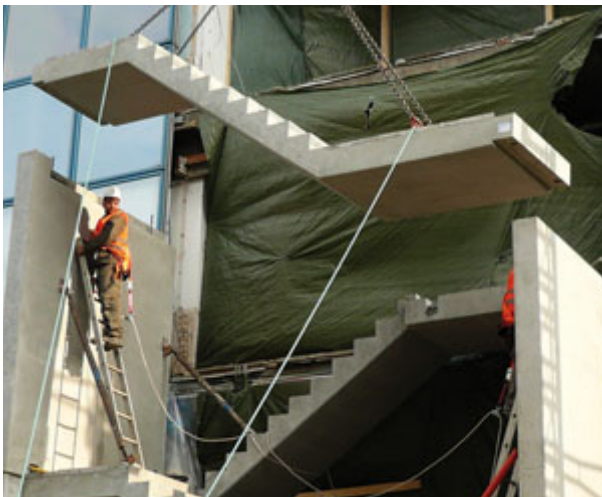
Fig. 7: Assembly of staircase flight including landings
