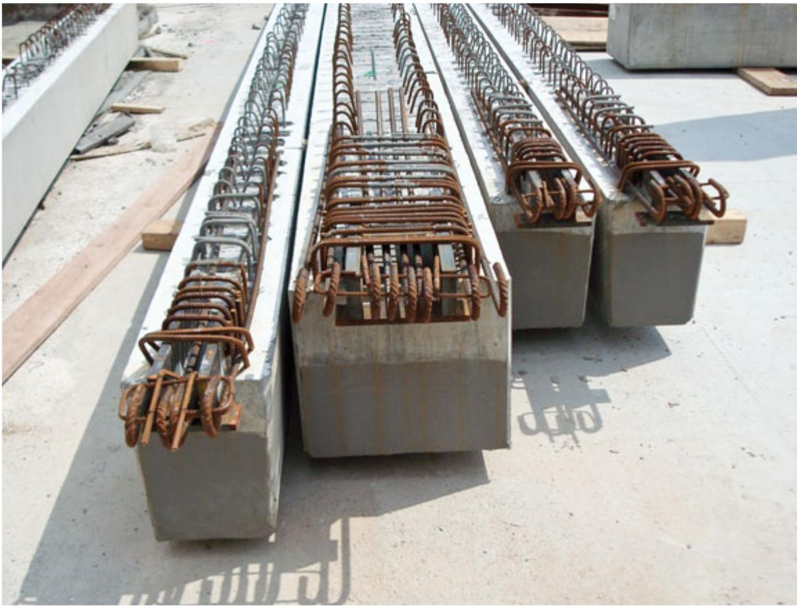
Fig. 6: Beam ends equipped by PBH Corbels
