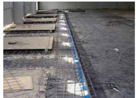
Figures 3 and 4: The straight and curved elements installed prior to pouring concrete.
