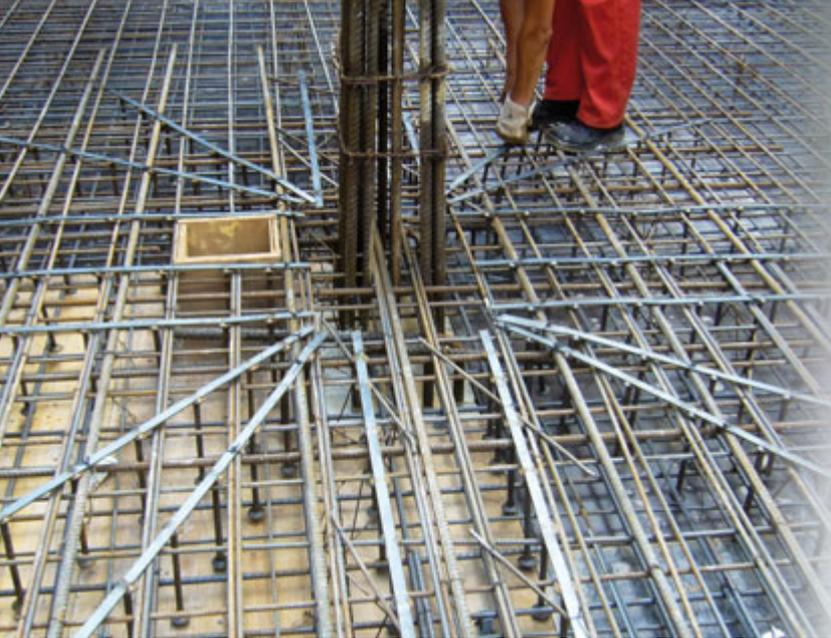
Figure 2: PSB punching reinforcement in formwork
